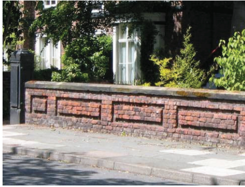
Low brick walls with recessed panel detail and a variety of coping stone
