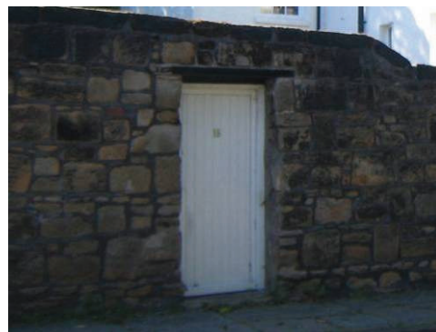
Simple boarded gateway in random rubblestone wall
