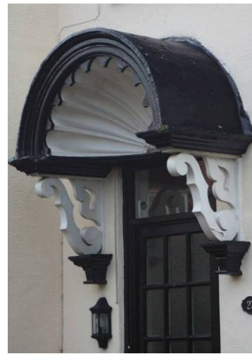
Shell porch canopy.
