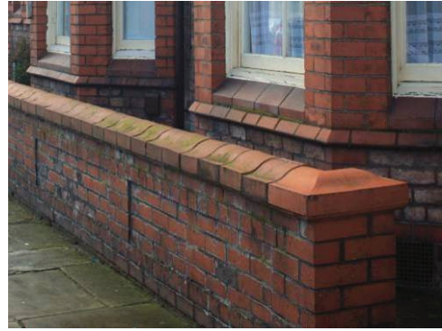
Low brick walls with recessed panel detail and a variety of coping stone
