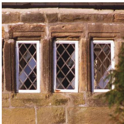
C17th sandstone 3-light ovolo moulded mullioned window, fitted with metal frames and leaded lights
