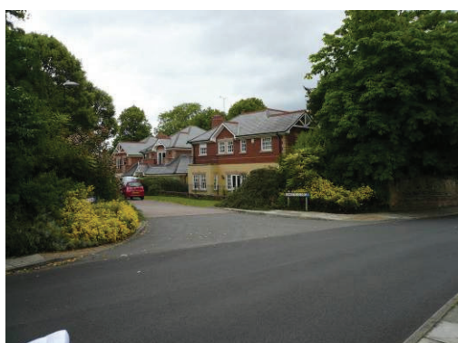
New Housing in Duncote Close
