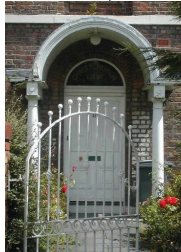
Late Georgian / Regency style door with elegant projecting porch canopy
