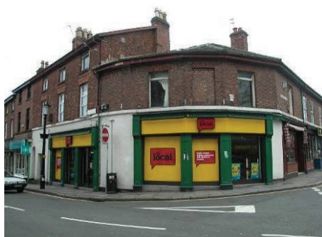
Poorly designed shopfronts, intrusive signage and gaudy colours on the corner of Christchurch Road and Claughton Firs undermine the historic townscape of the village centre.
