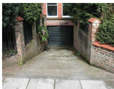
Basement converted to garage on Village Road
