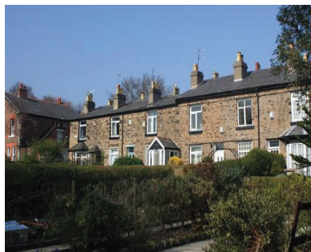
Salem View from the east/west, which is the southernmost point of the conservation area (Dxxx SAL-VW)
