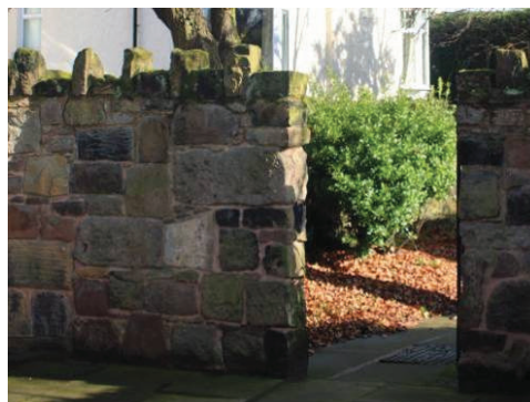
Example of 'cock and hen' coping, which adds variety to the streetscape
