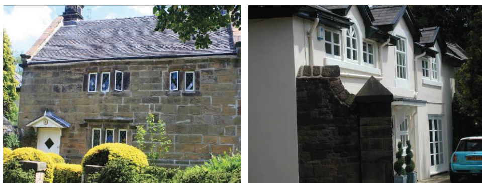
Oxton Old Hall and converted stable buildings off Talbot Road
