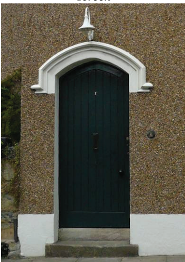
Gothick style vertical boarded door with simple hood mould externally
