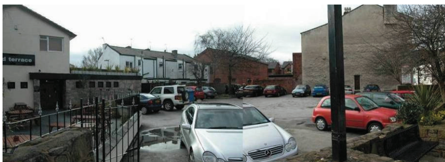
Loss of enclosure around car park at village centre
