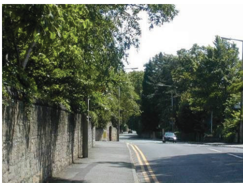
View south along conservation area boundary adjoining Talbot Road (D881 TAL-RD)
