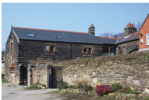
Vernacular buildings on Newburns Lane
