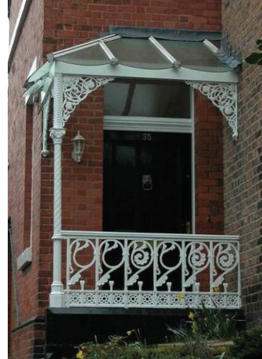
Six panelled door to wrought iron traceried balcony
