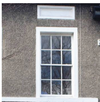
Conventional 12-pane double-hung sliding sash window with fine glazing bars in rectangular opening, given additional character by recessed panel above and projecting cill band below
