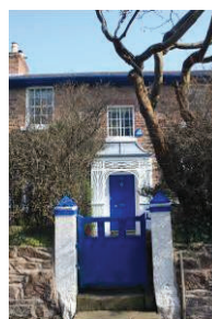
14 Fairview Road (listed)
