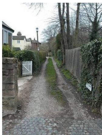
South Bank, where stone sets and rammed stone make an attractive surface.
